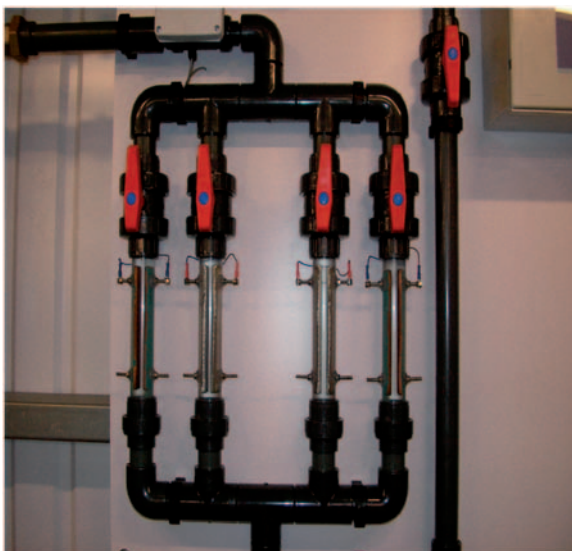
Figure 3. Copper–silver ionization system showing two copper and two silver electrodes
