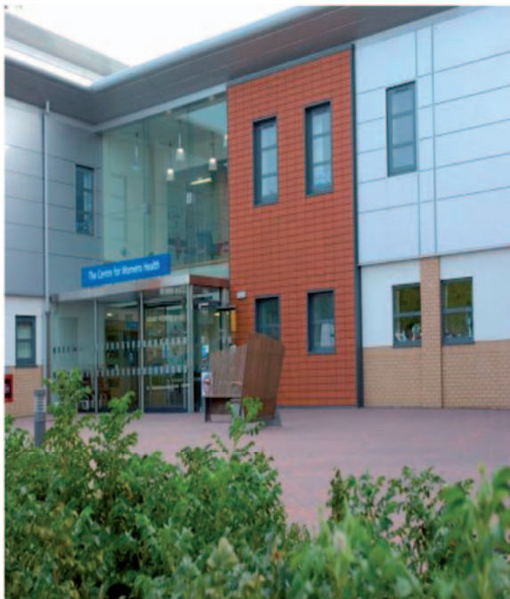
Figure 1. The new maternity–gynaecology extension
