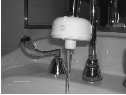
Plate 1.5 Outlet with point-of-use water filter attached (Sheffer et al. , 2005)
