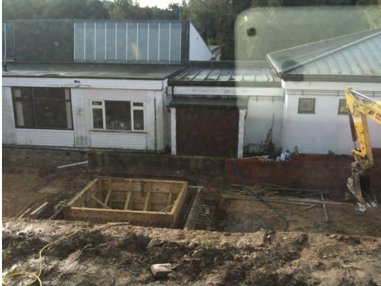
Plate 3.3 Study hospital 9 – photograph of construction work started in May 2010.
