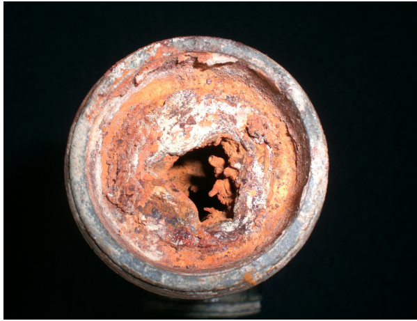
Plate 1.4. Inner surfaces of an eroded galvanized pipe. (ProEconomy Ltd, 2006)
